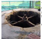
The picture is of the existing cast iron 'cross tree' which is to be replaced with stainless steel. This steelwork supports the 'holding down' rod which keeps the spire under compression. Amazing!
